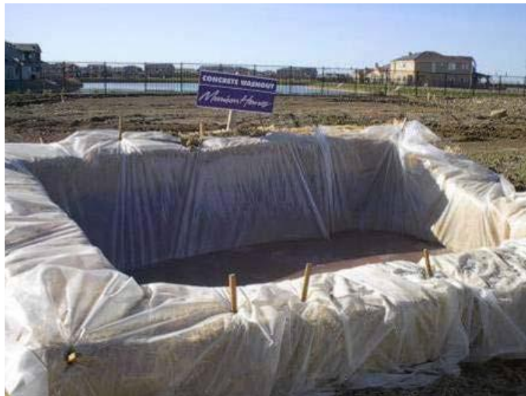
Plate 2.1: Example of a Temporary Concrete Washout Area
